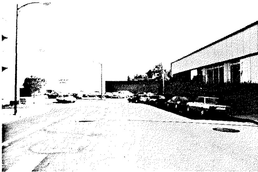
Figure 12: Existing View Along Broadway Plaza
