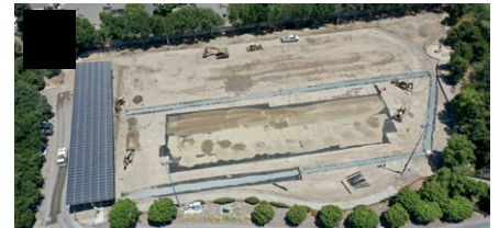
CREWS WORK TO GRADE AND BUILD UP THE BASE SURFACE. DRAINAGE IS IMPORTANT
